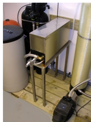
Mach 4060⇒TC 401c⇒Tank⇒Pump⇒Neutralizer
