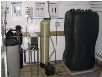
Mach 4060⇒TC 401c⇒Tank⇒Pump⇒Neutralizer
